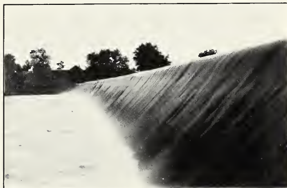
DUNDEE DAM, PASSAIC RIVER. One Mile Above Passaic.
